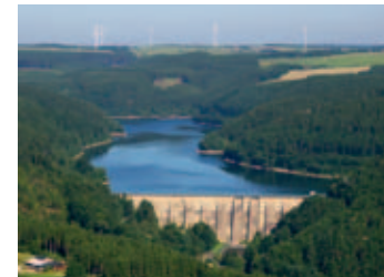
City water supply
